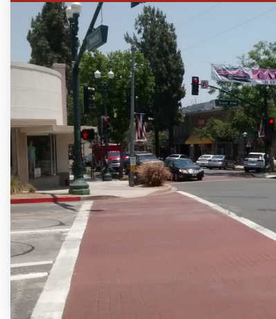
Textured pavement at Montrose and Honolulu in Glendale Photo from Nelson\Nygaard
