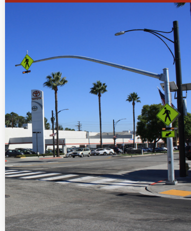
RRFB in Glendale Photo from the City of Glendale
