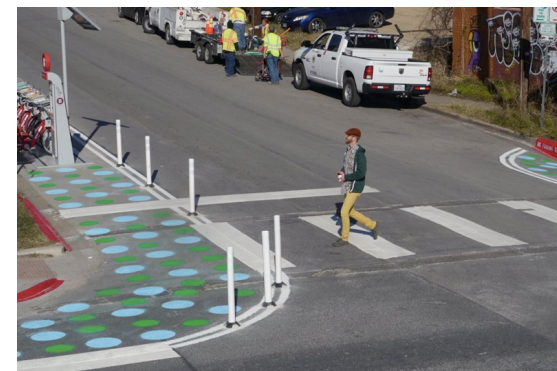
A temporary, low-cost curb extension in Austin, TX Image from Austin Mobility
